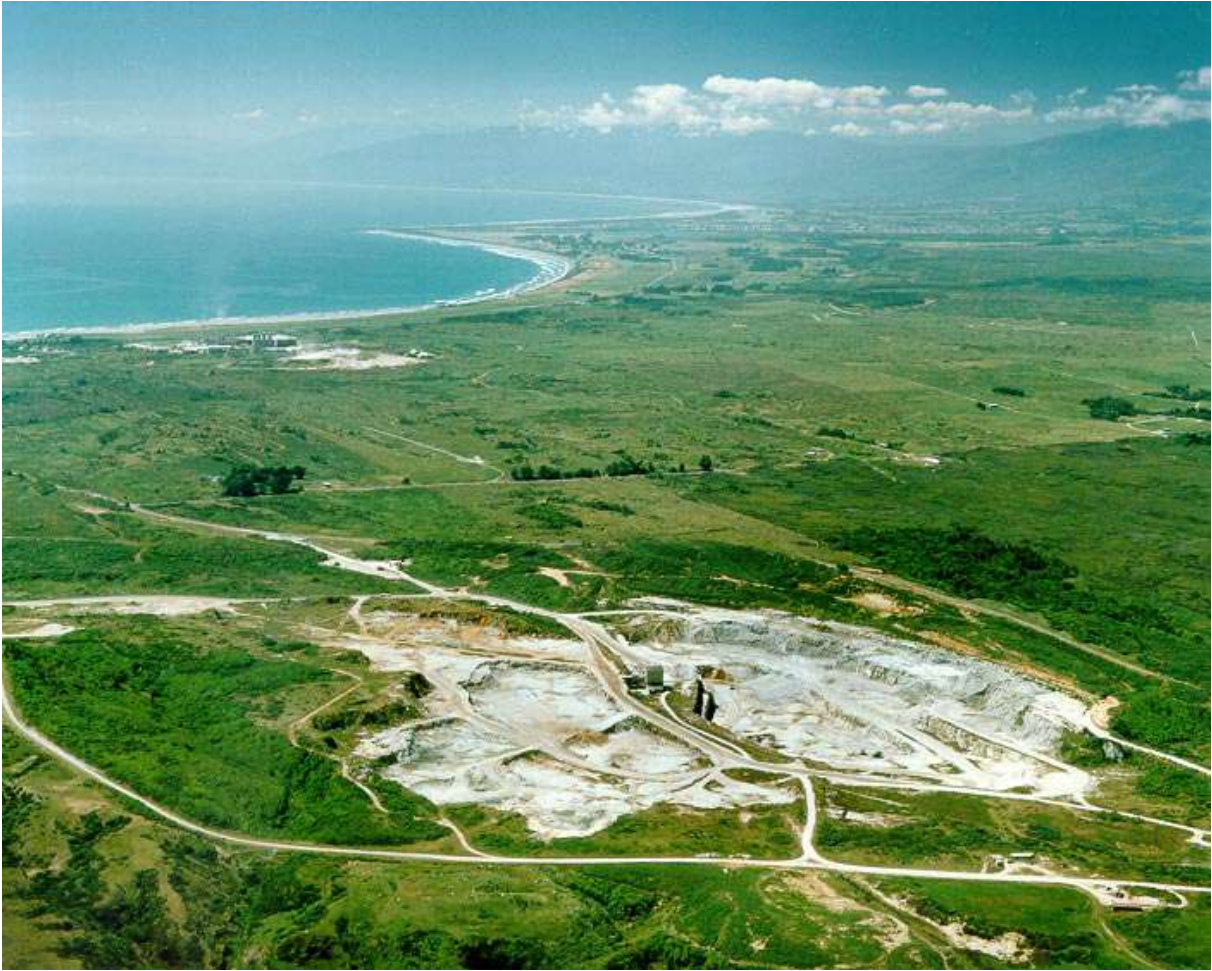
Figure 30 Cape Foulwind Limestone quarry (foreground), cement plant (middle distance), and Westport (far distance) (GNS photo, photographer Lloyd Homer).
