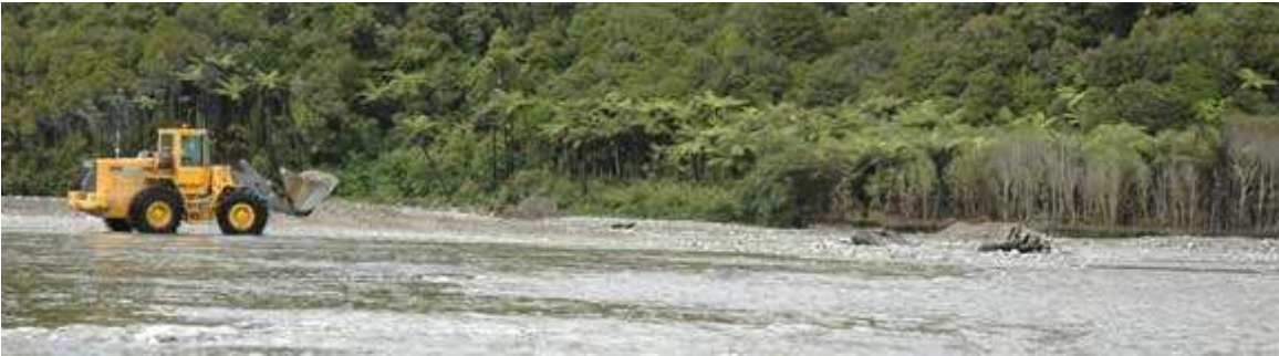
Figure 24 Mining river gravel for aggregate (photo courtesy of Minerals West Coast).
