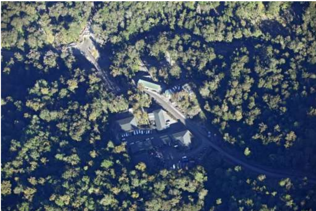
Figure 47 Pike River mine building blended into native bush (May 2009 photo courtesy of Pike River Coal Ltd).
